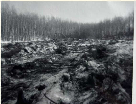
CLEARING SPORTS AREA
