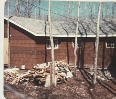
H- HUT NEARING COMPLETION
